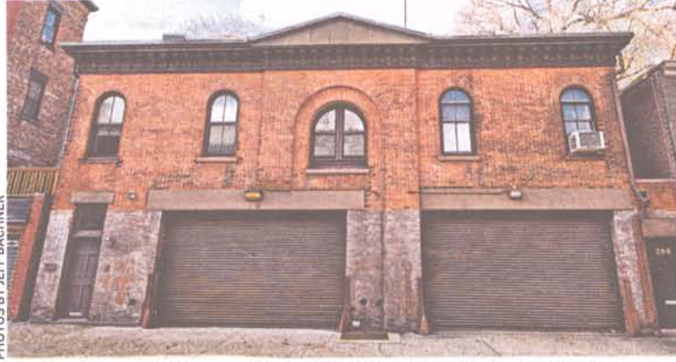
Carriage houses, like this one at 266 Waverly Ave., are common in Clinton Hill
